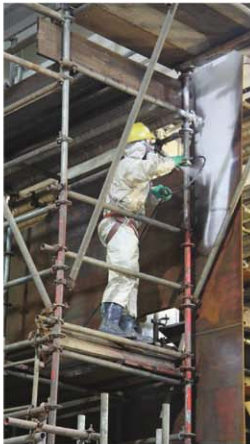
Application of first system coat after UHP waterjet-cleaned surface.
