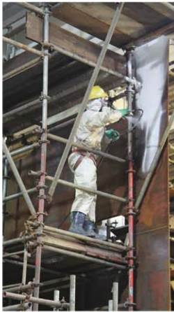
Application of first system coat after UHP waterjet-cleaned surface.
