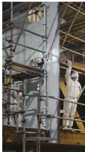
Third and final system coat being applied.
