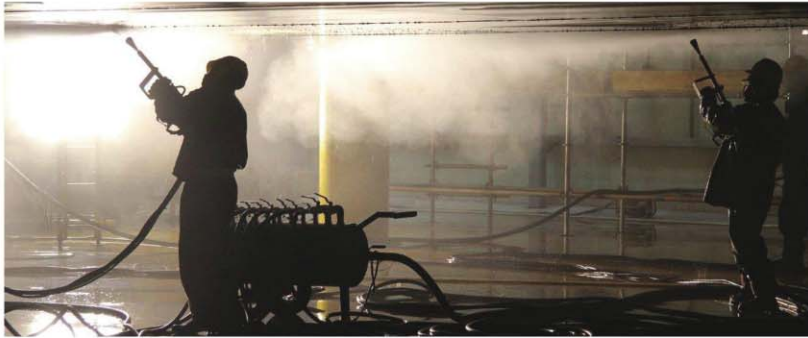
Workers being trained in UHP waterjetting operation.
